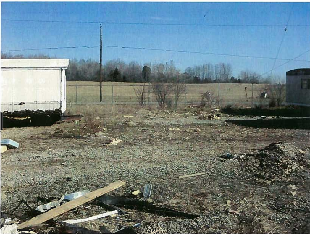
Date: 03/13/2012 Time: 9:57 a.m. Direction: north Photo by: Garrison Gross Exposure #: 004 Comments: scattered debris
